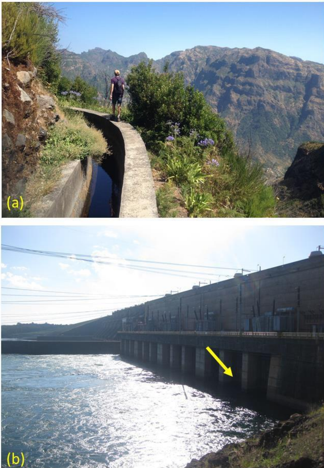
Figure 3. (a) A channelized concrete levada on the island of Madeira. (b) The arrow shows the tailrace of the Igarapava Dam, Brazil.
